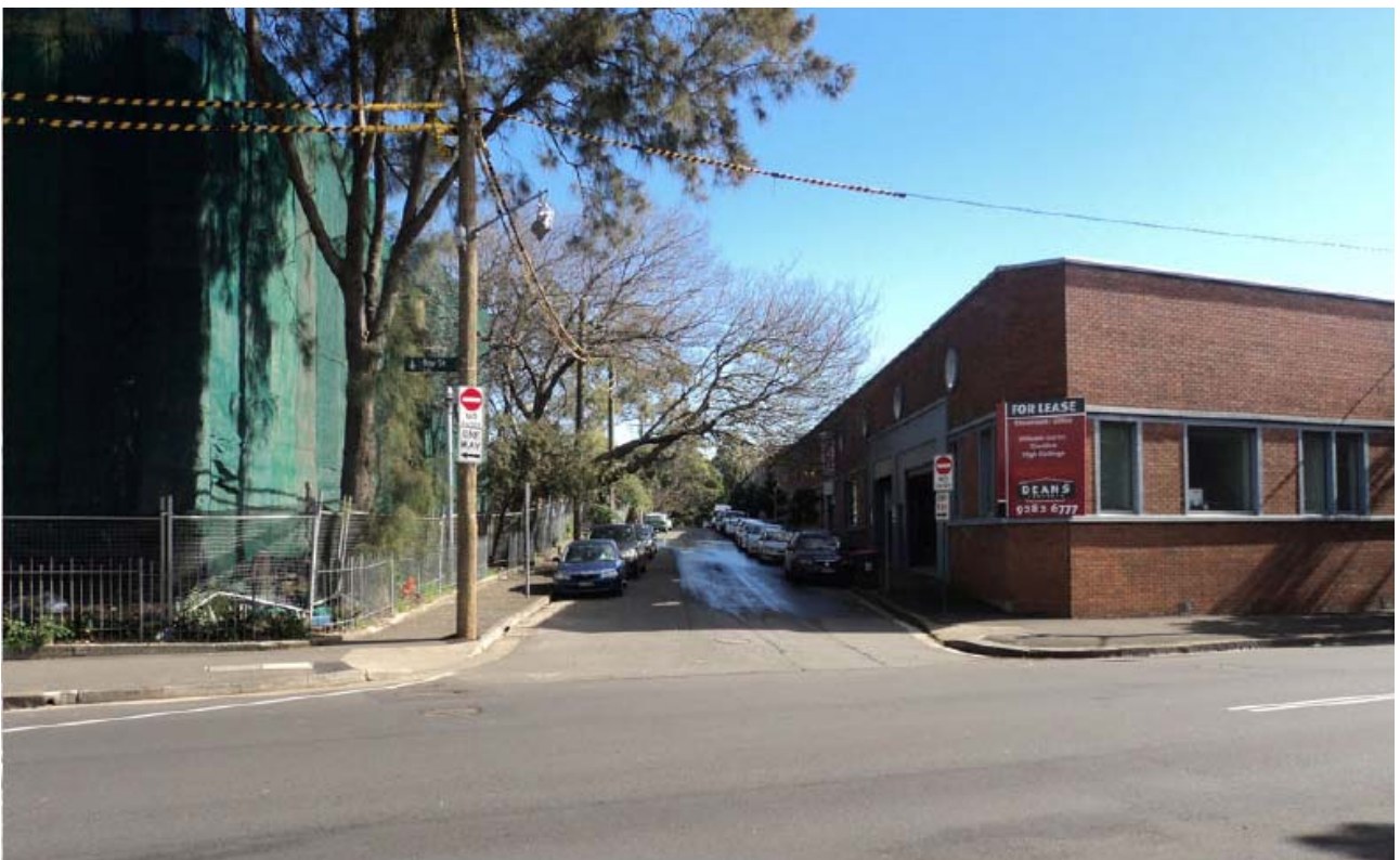
Figure 4: Rear of existing development, taken from the Bay Street, looking down Wentworth Street.
